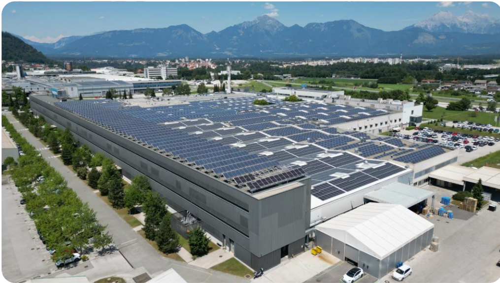
Kranj: Iskra BU MIS Solar power plant
