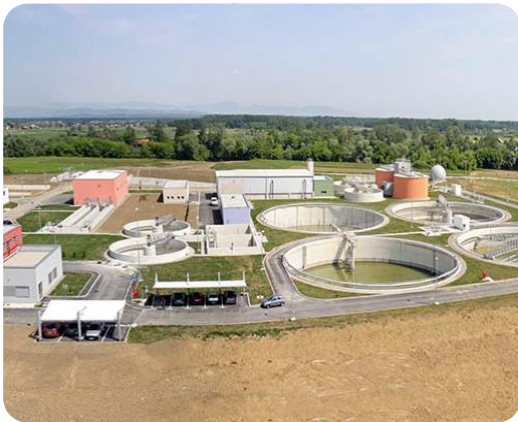
Karlovac - Croatia: WWTP
